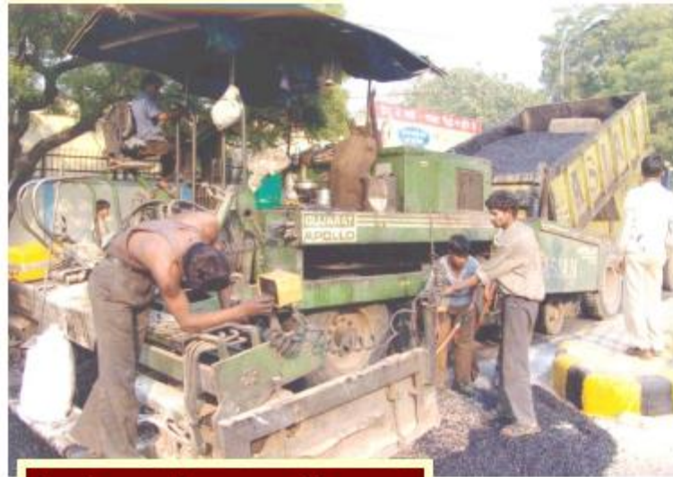
Laying and compaction
